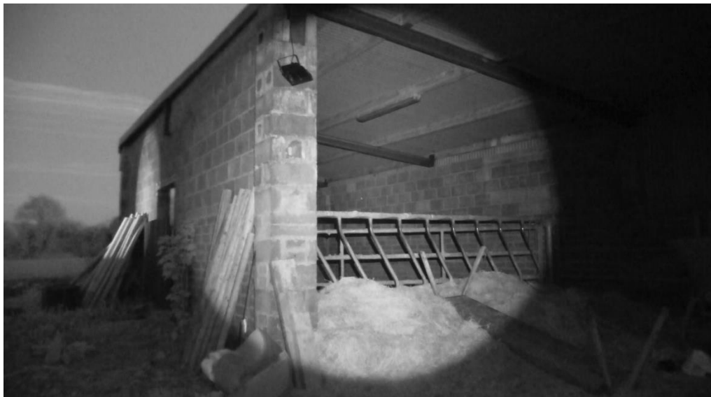
Plate 0-2: 5 Structure 2 – Shed next to Dwelling, 1 Bat emerged.
